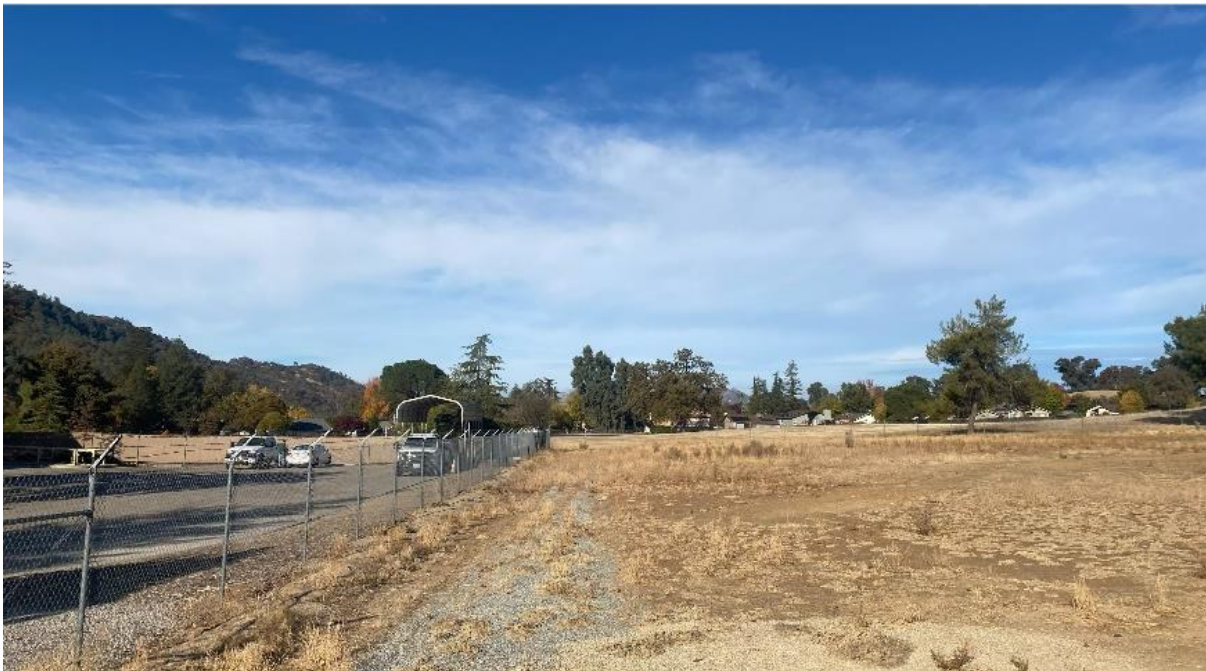
Photograph 2. Photograph of existing wastewater treatment plant facilities and Action Area, facing northwest. November 22, 2024.
