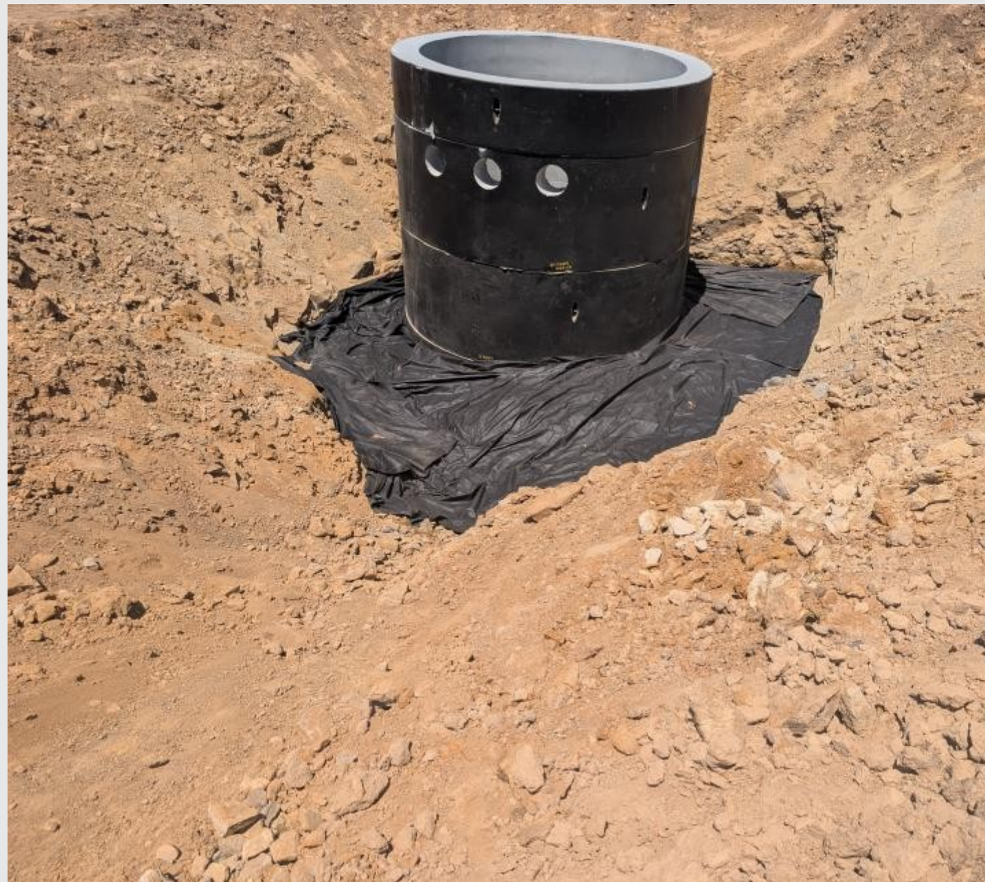
Influent Lift Station Install
