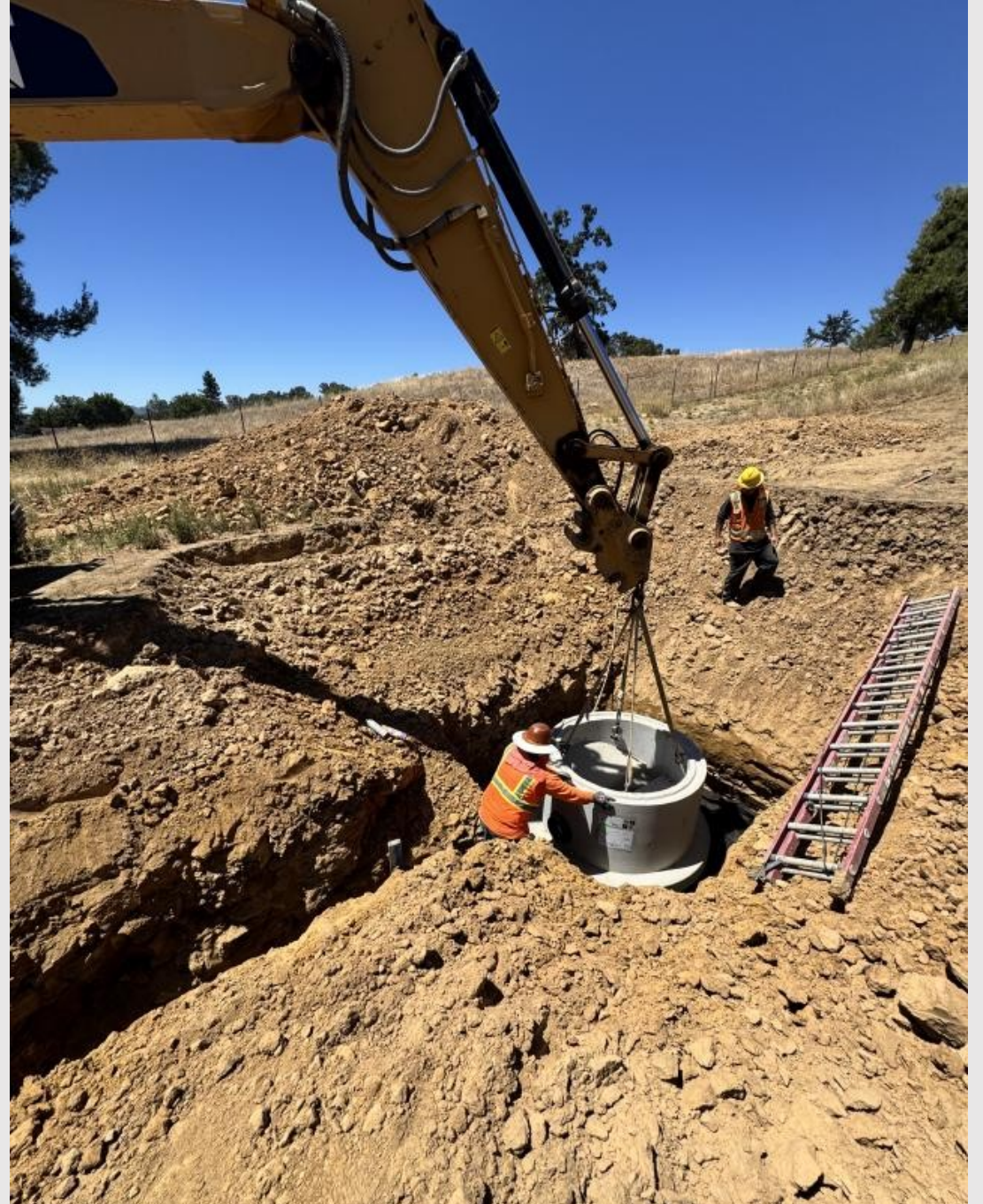
Set bases for CB-1 and 2 and Pond 1 MH
