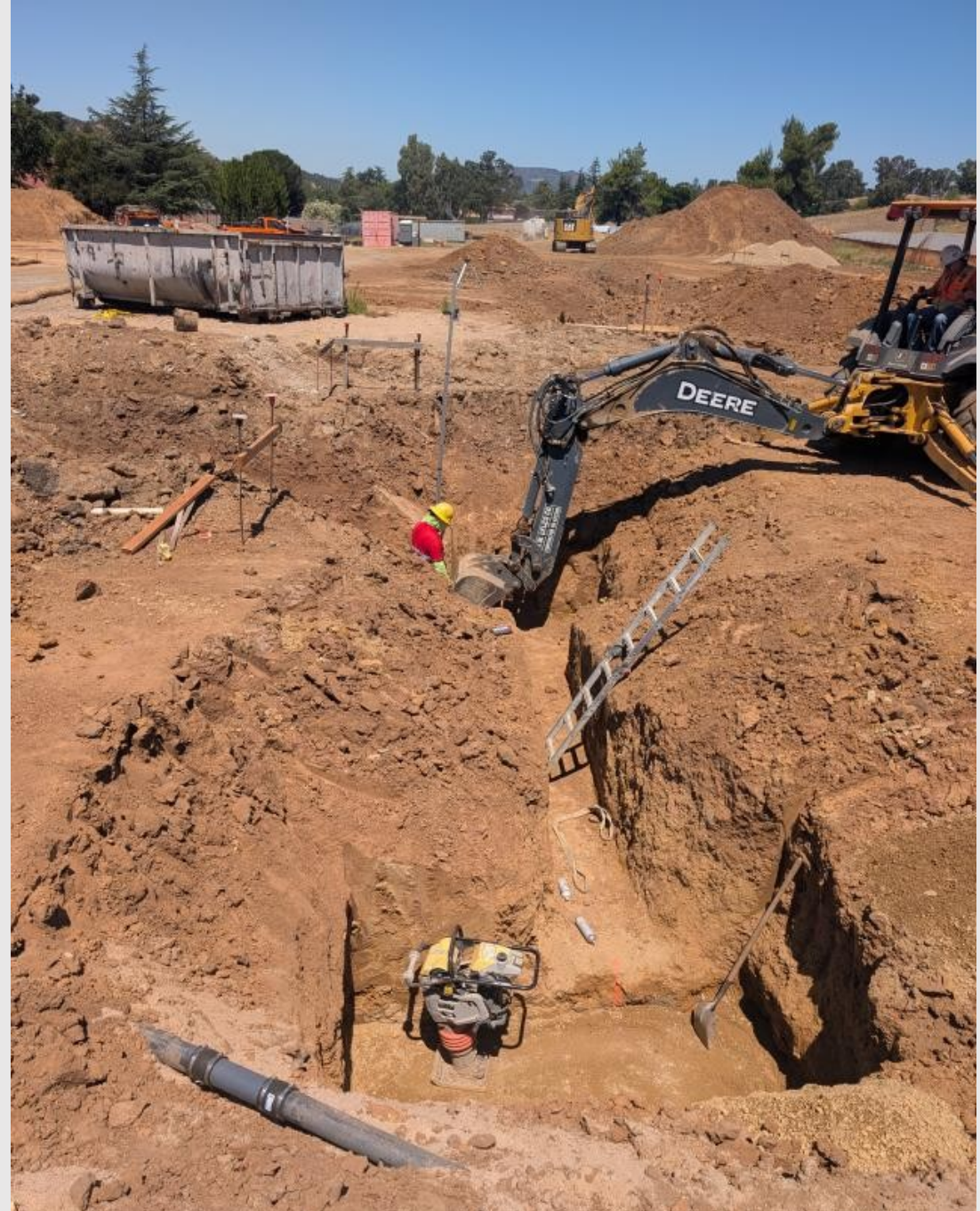
Trench for catch basins and under slab pipes
