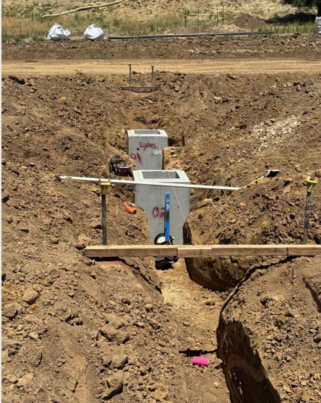
Set bases for CB-1 and 2 and Pond 1 MH
