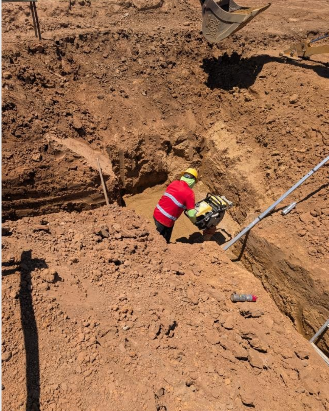
Trench for catch basins and under slab pipes
