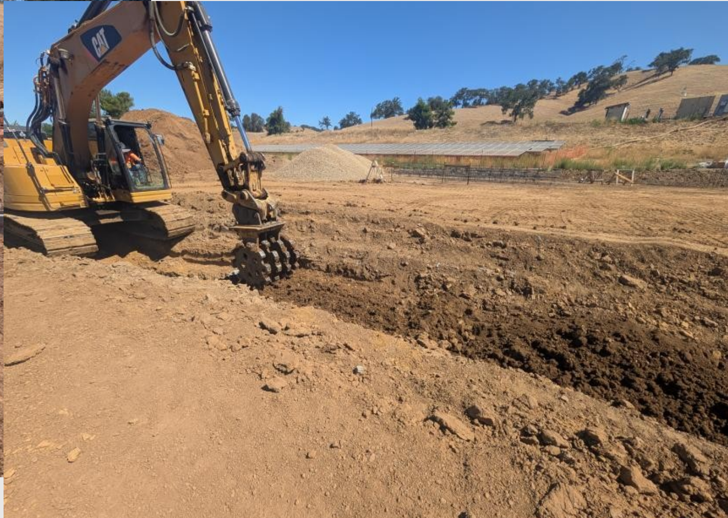
Backfilling and compacting
