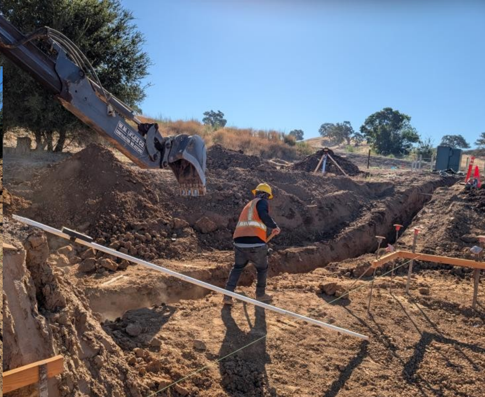
Trench for PGE main feed
