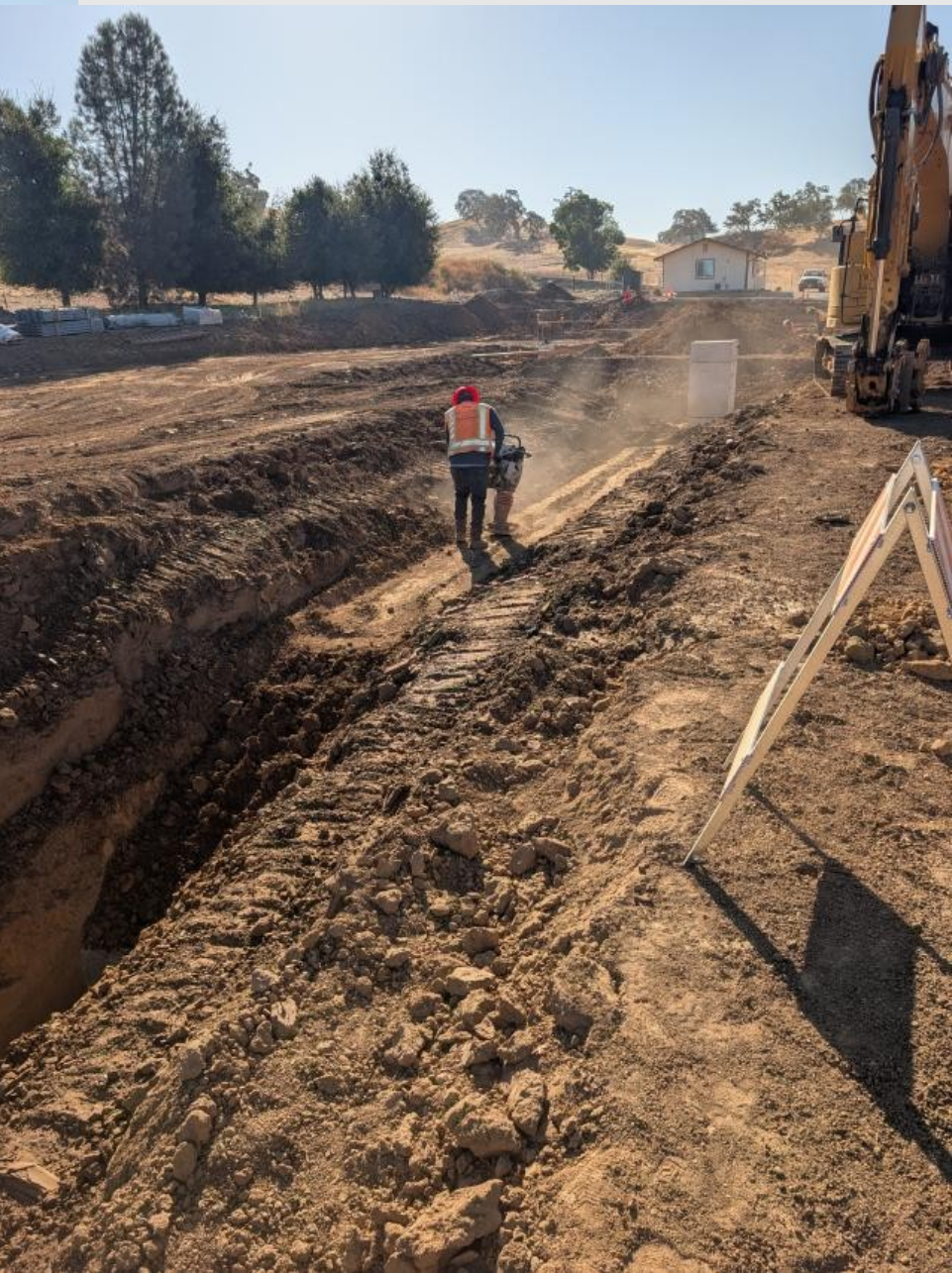
Backfilling and compacting
