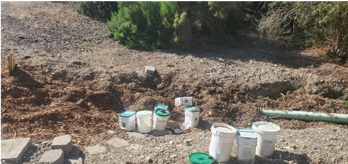
Photograph 4. Photograph of the de-chlorination process replacement location at the spray field, facing west. October 6, 2022.
